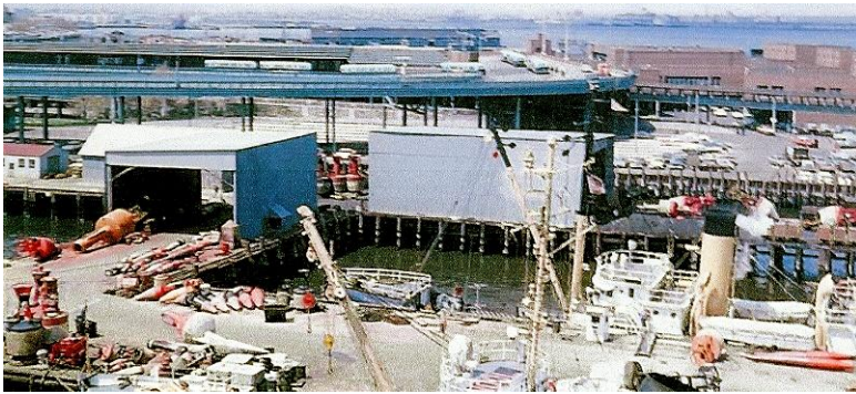
#B-37, looking toward Ferry Terminal St. George.
